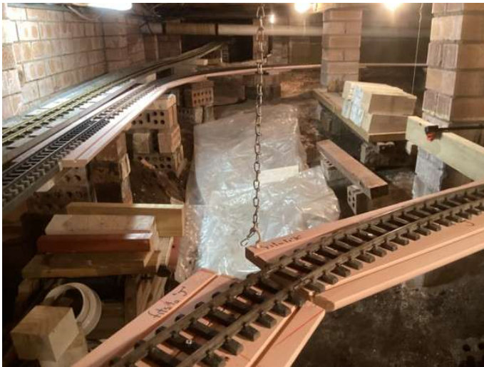
Chain is attached to a screw hook until a base pad can be installed and levelled below. Prop has since been placed.
