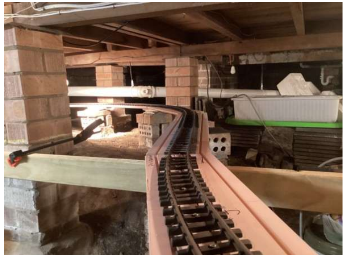
Horizontal bearer to support curve and straight transition.
