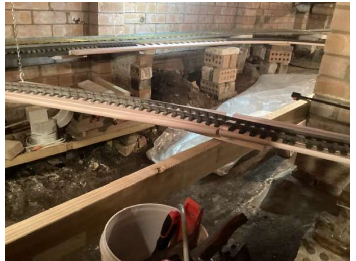
Once all the supports were levelled with packers, it took less than ten minutes to fit all the arc pieces.
