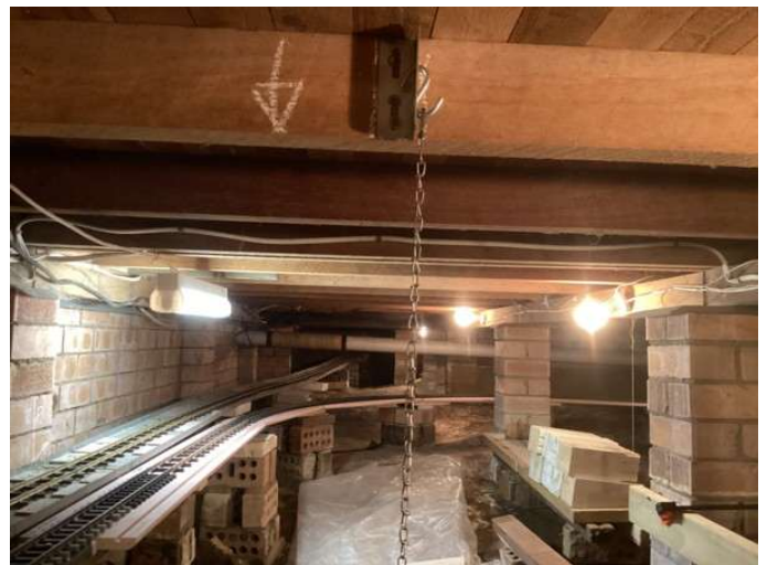
Chain is temporary until a prop can be founded below.
