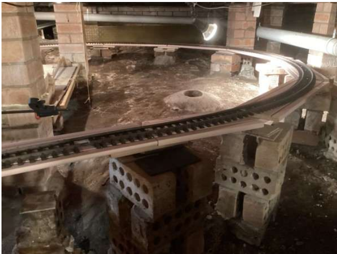
Once all the supports were levelled with packers, it took less than ten minutes to fit all the arc pieces.
