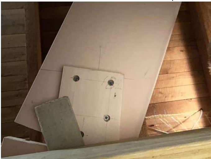
Screws are under track base boards in each Splice plate and are screwed to the clockwise end of each arc only, this allows dismantling some time in the future.
